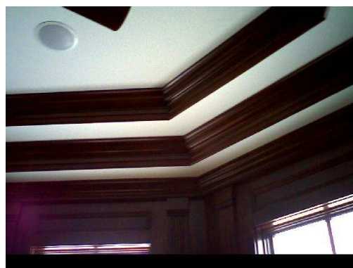
Soffit area main office over windows. Lower tier.
