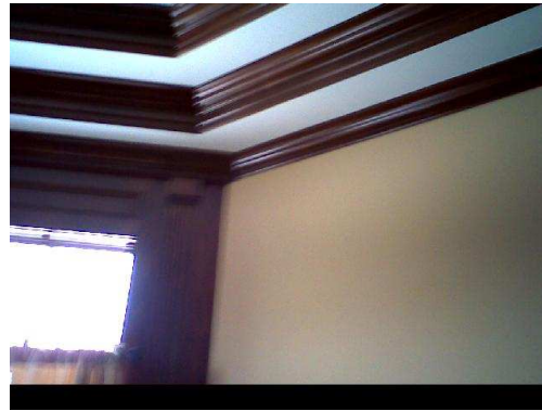
Main office right wall from entry door view.
