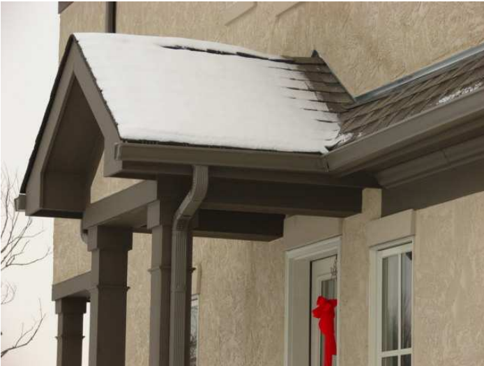
Dormer/porch cover on side of house
