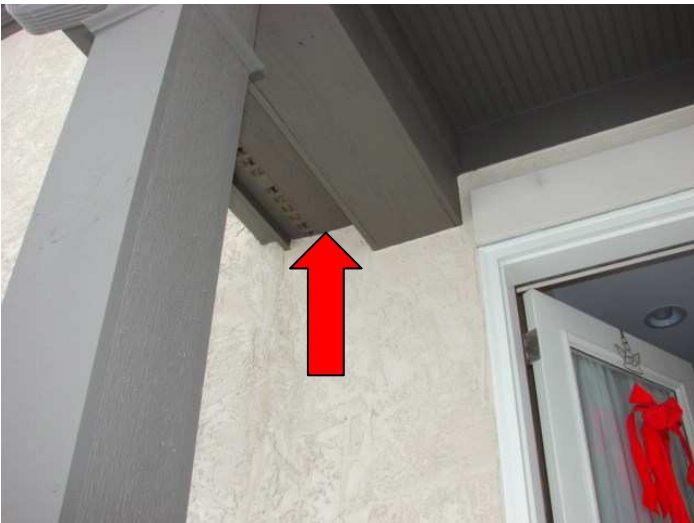
Areas of concern at dormer/porch cover soffit vents
