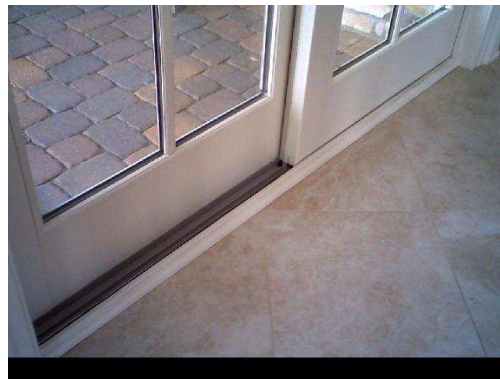
Sliding door on right side of eating area to porch.
