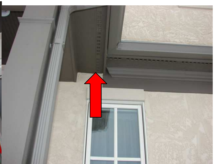
Areas of concern at dormer/porch cover soffit vents
