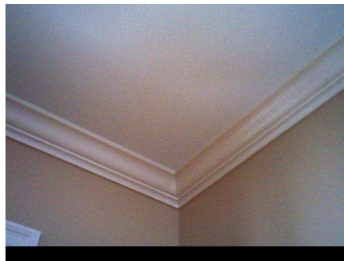
Soffit in front right corner of main dining room.
